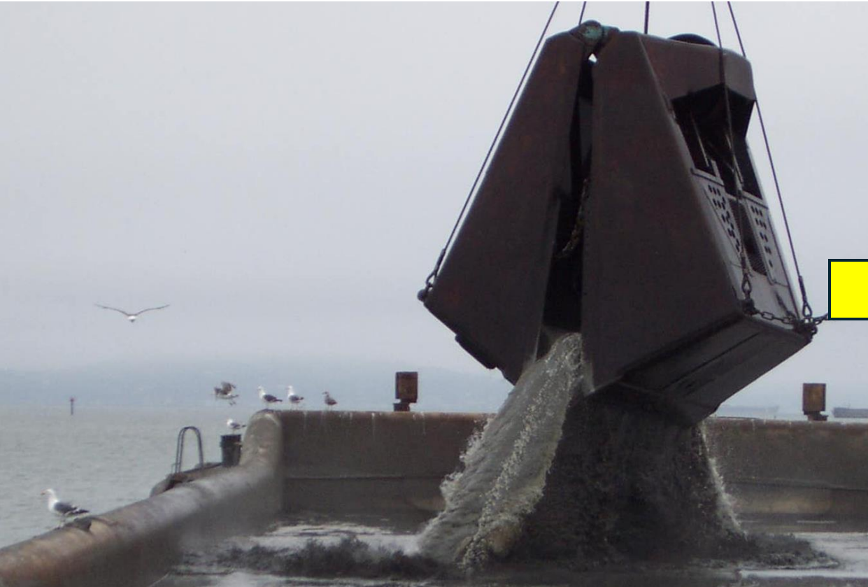
Sediment dredged from Bay, streams, channels
