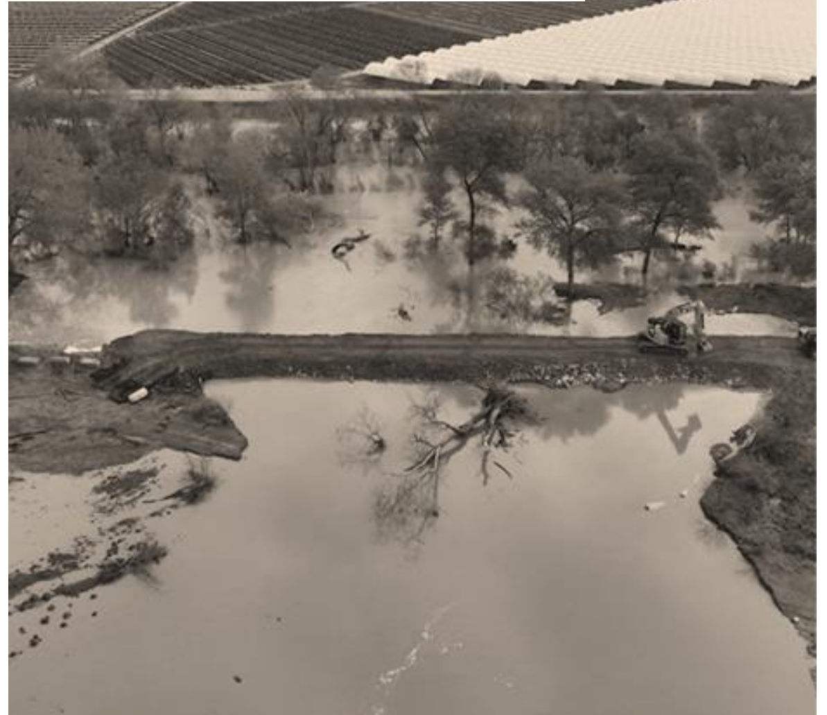
Pajaro River levee, Monterey County
