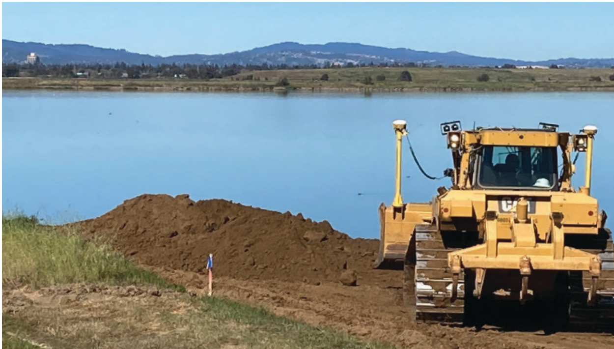
▲ Upland soil being being beneficially reused at south bay salt ponds. Credit: Dave Halsing
