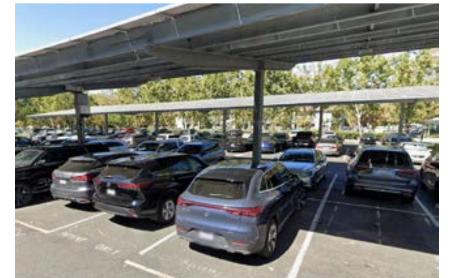
SIMILAR SOLAR STRUCTURES IN FREMONT, CA
