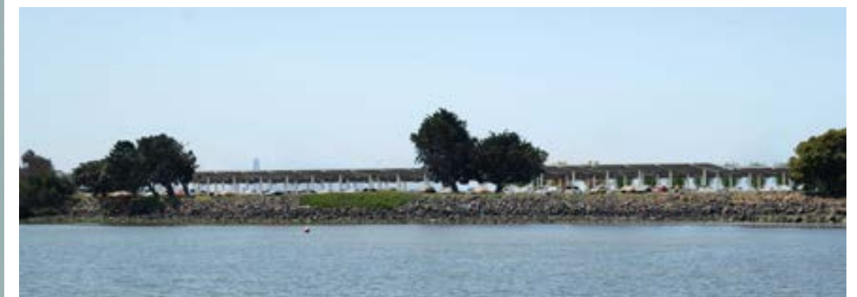
5 Future solar panels
