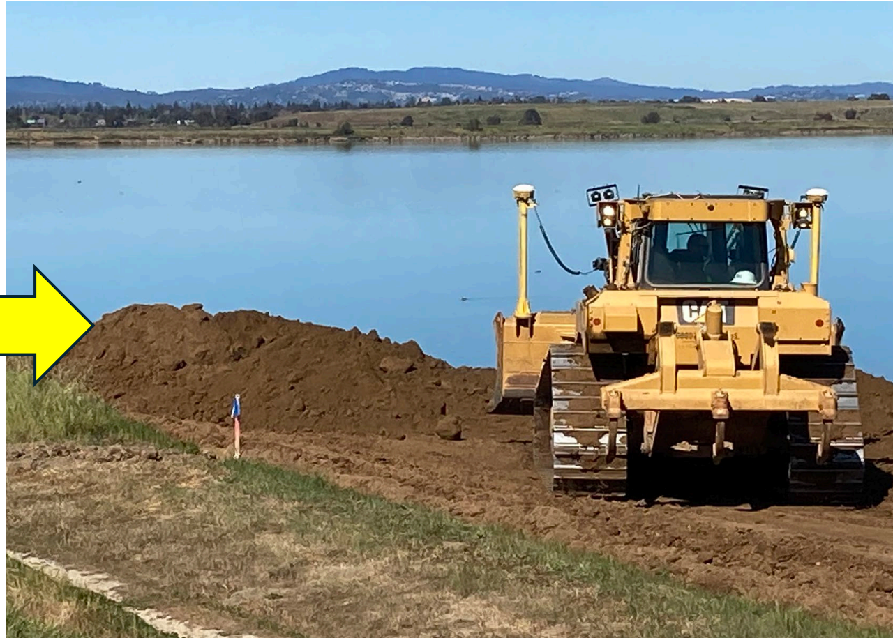
Soil reuse at South Bay Salt Ponds Restoration Project
