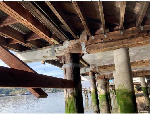
Figure 2. Image showing some new pilings and a portion of the new deck.
