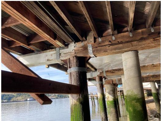
Figure 2. Image showing some new pilings and a portion of the new deck.
