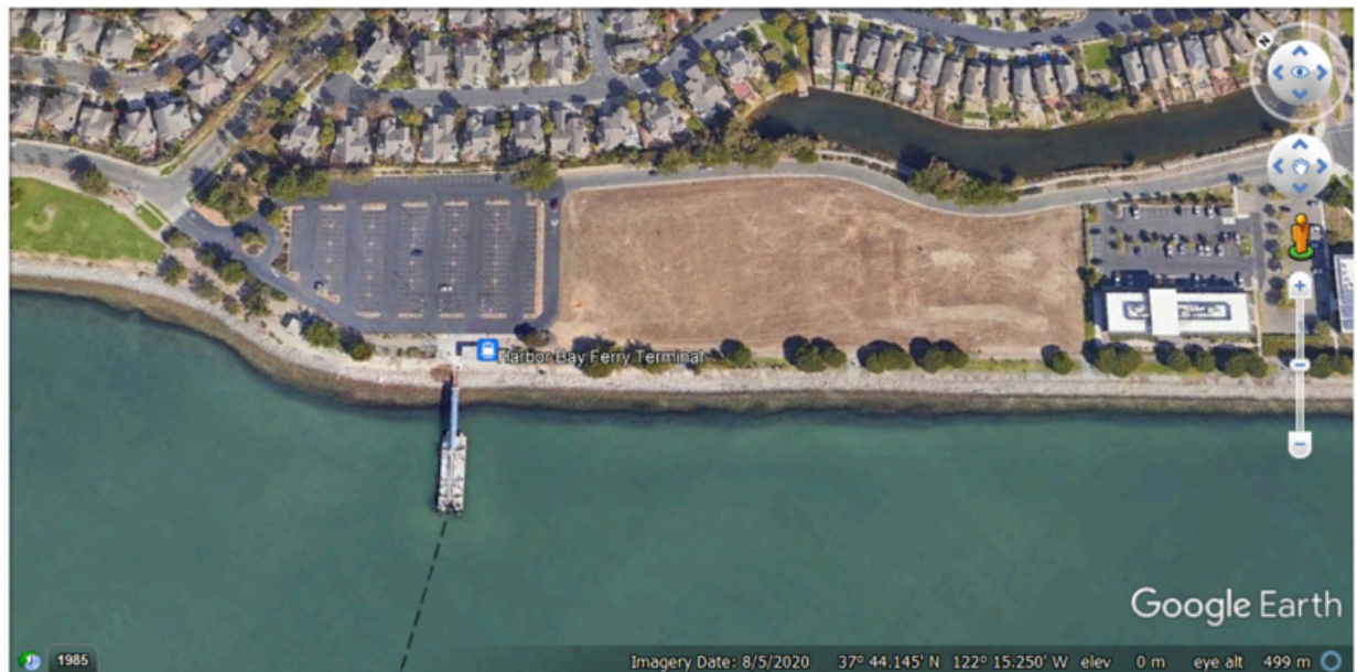
Above: WETA Harbor Bay ferry terminal in a modern residential development devoid of historical and existing recreation. The City of Alameda offers parking for 250 cars and two motorcycles at this terminal.
