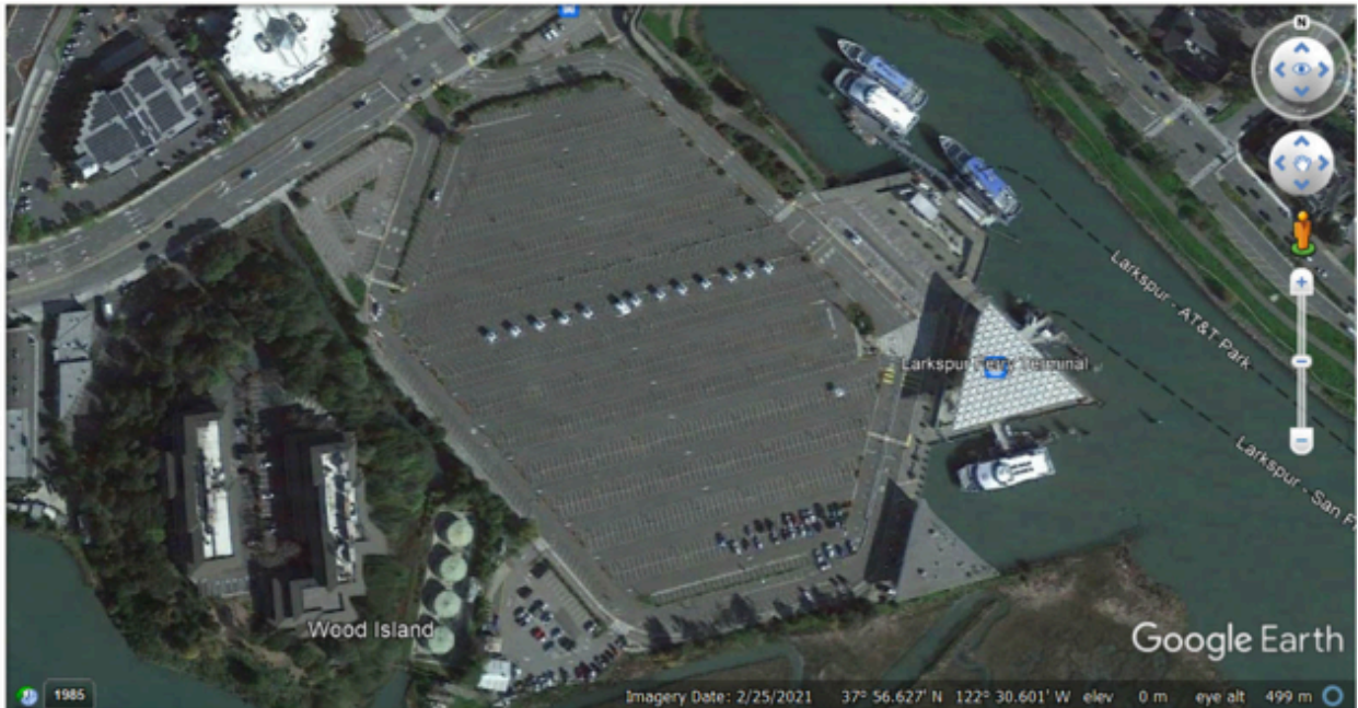
Above: Larkspur Landing Golden Gate ferry terminal with 1800 parking spaces. This was taken during covid when the lot was empty.
