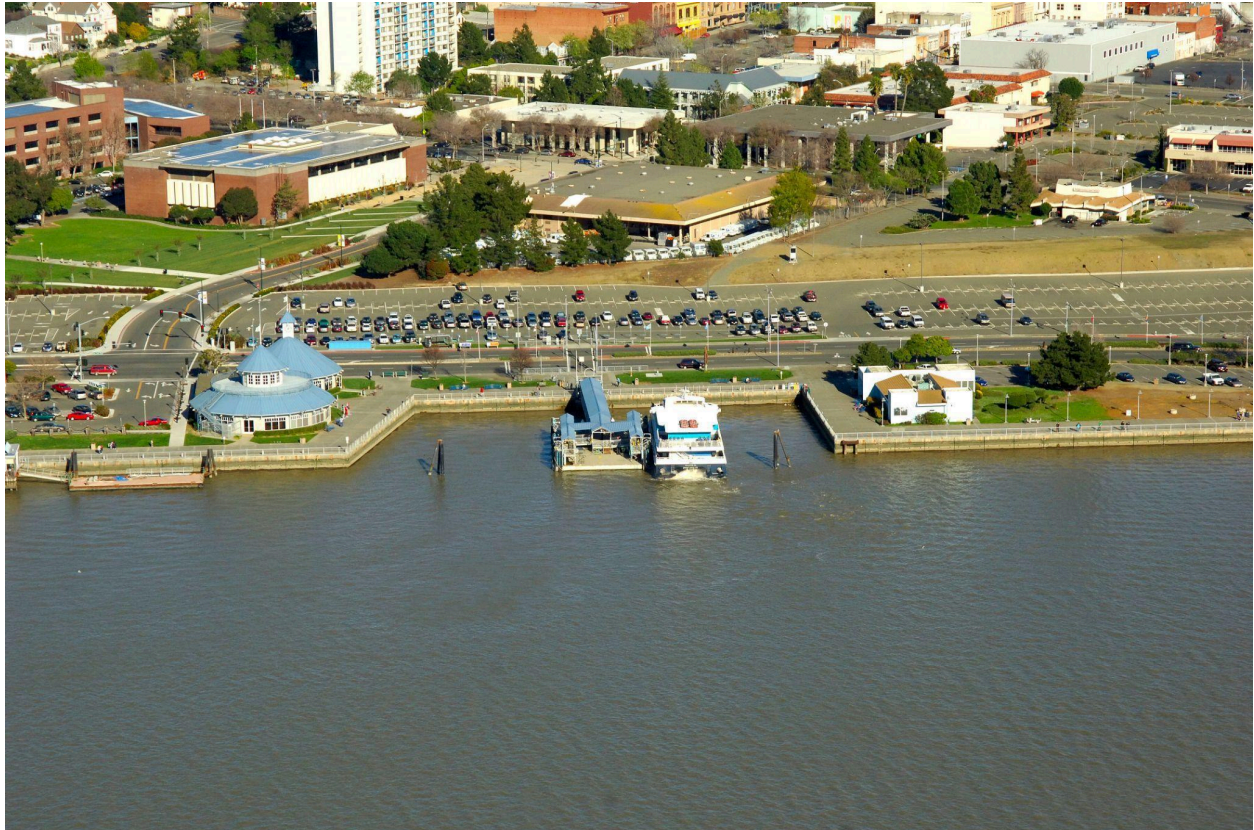
Above: WETA Vallejo ferry terminal. There is a waterfront parking garage and several surface lots directly across from the ferry terminal that serve ferry commuters. These include the City of Vallejo's waterfront garage plus multiple adjacent public lots. Over ~750+ spaces are available in the waterfront parking garage and surface lots near the ferry terminal combined (for daily paid parking). The main waterfront garage and the adjacent surface lots across from the Vallejo Ferry Terminal require payment (around $8 per 24 hours or a $50 monthly pass) for ferry patrons and other users. There are five paid parking lots available around the Vallejo Ferry Building which have security regularly patrolling the lots. Source: Vallejo Ferry Parking map .
