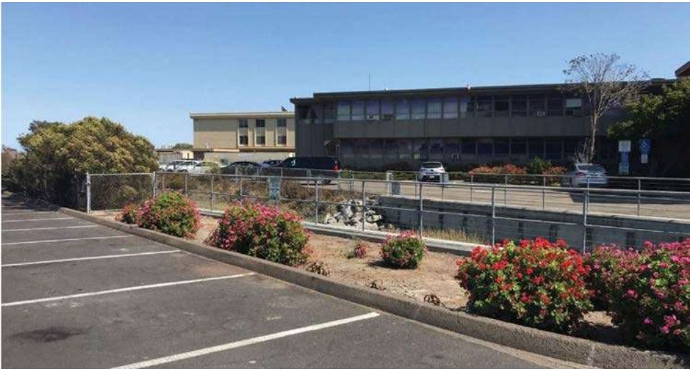
Easton Creek Culvert at Old Bayshore Highway
