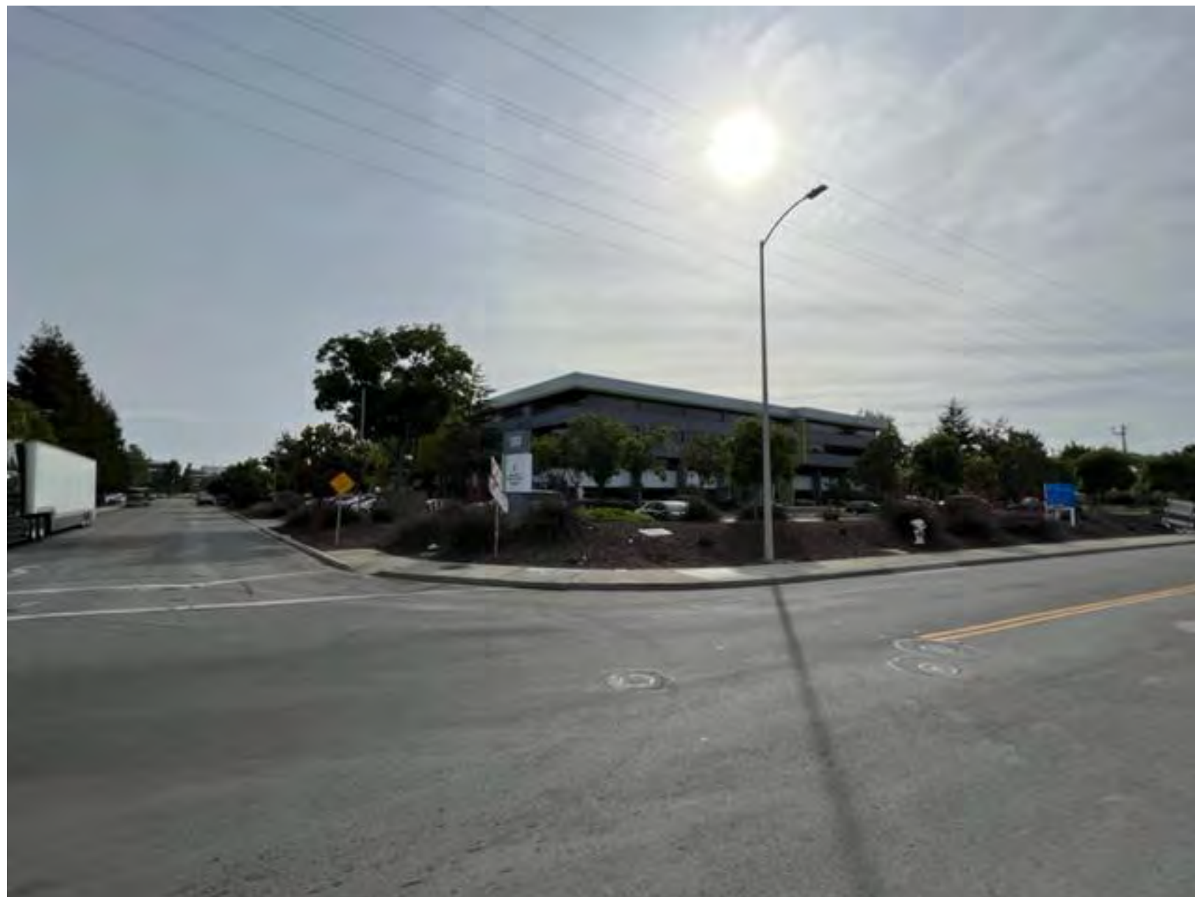
1 VIEW OF (E) 4 STORY BUILDING INTERSECTION OF SHOREWAY ROAD & SEM LANE - LOOKING EAST
