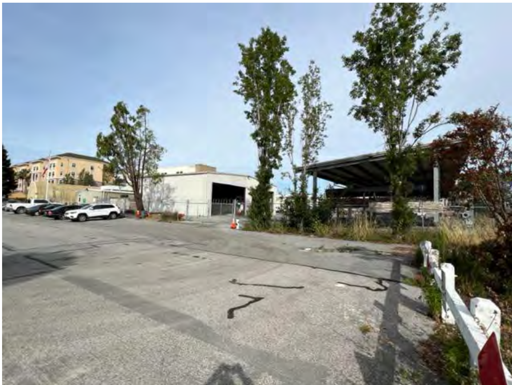
5 ADJACENT PROPERTY (CITY CORPORATION YARD) END OF SEM LANE @ BELMONT CREEK - LOOKING WEST
