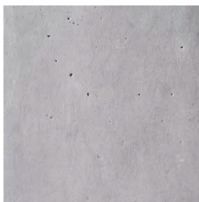
8 ARCHITECTURAL CONCRETE CAST-IN-PLACE
