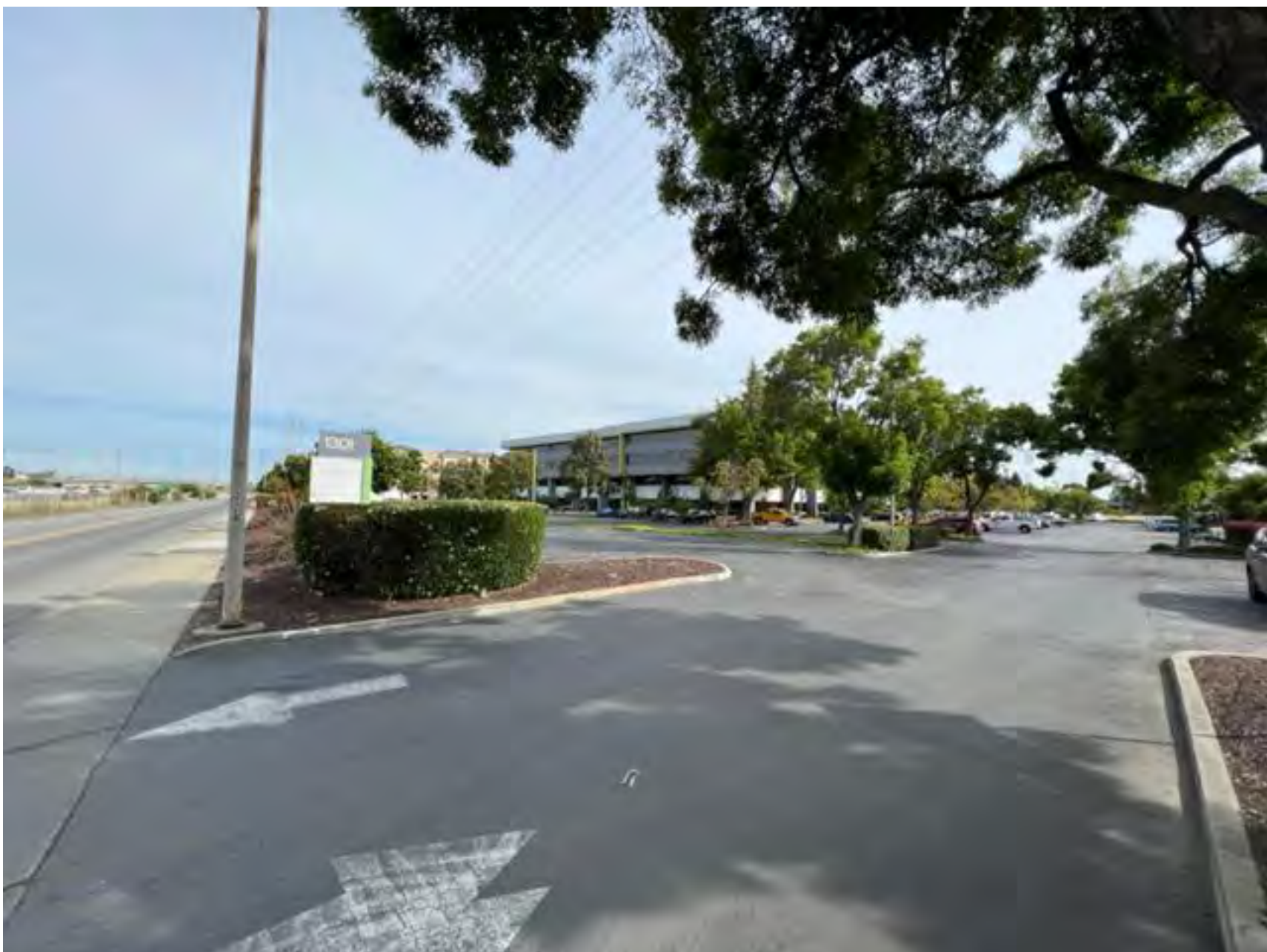
6 VIEW OF (E) 4 STORY BUILDING SITE ENTRANCE OFF OF SHOREWAY ROAD - LOOKING NORTH
