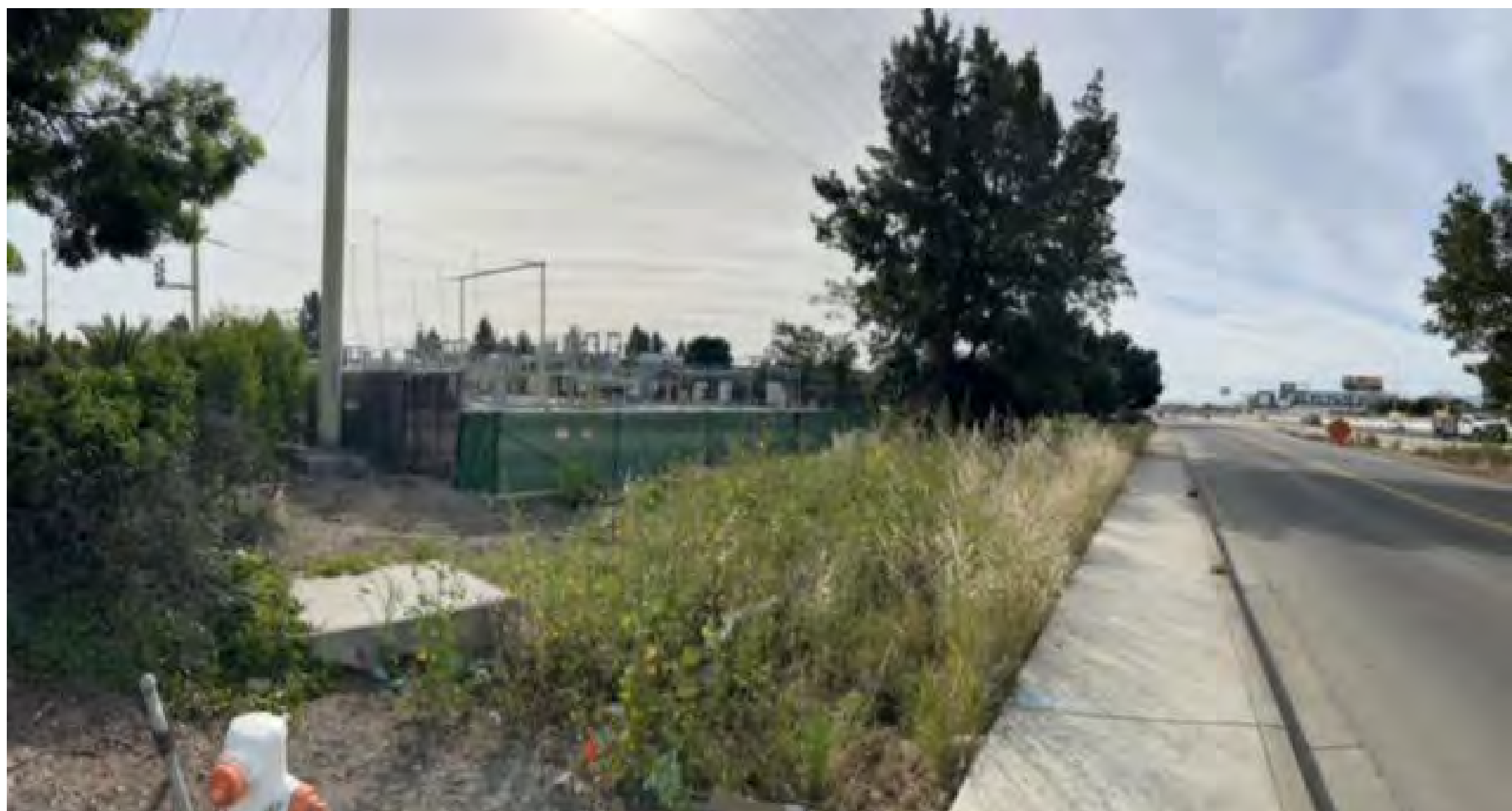
7 VIEW OF ADJACENT PROPERTY (PG&E) SITE ENTRANCE OFF OF SHOREWAY - LOOKING EAST
