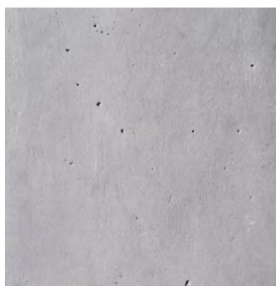
8 ARCHITECTURAL CONCRETE CAST- IN-PLACE
