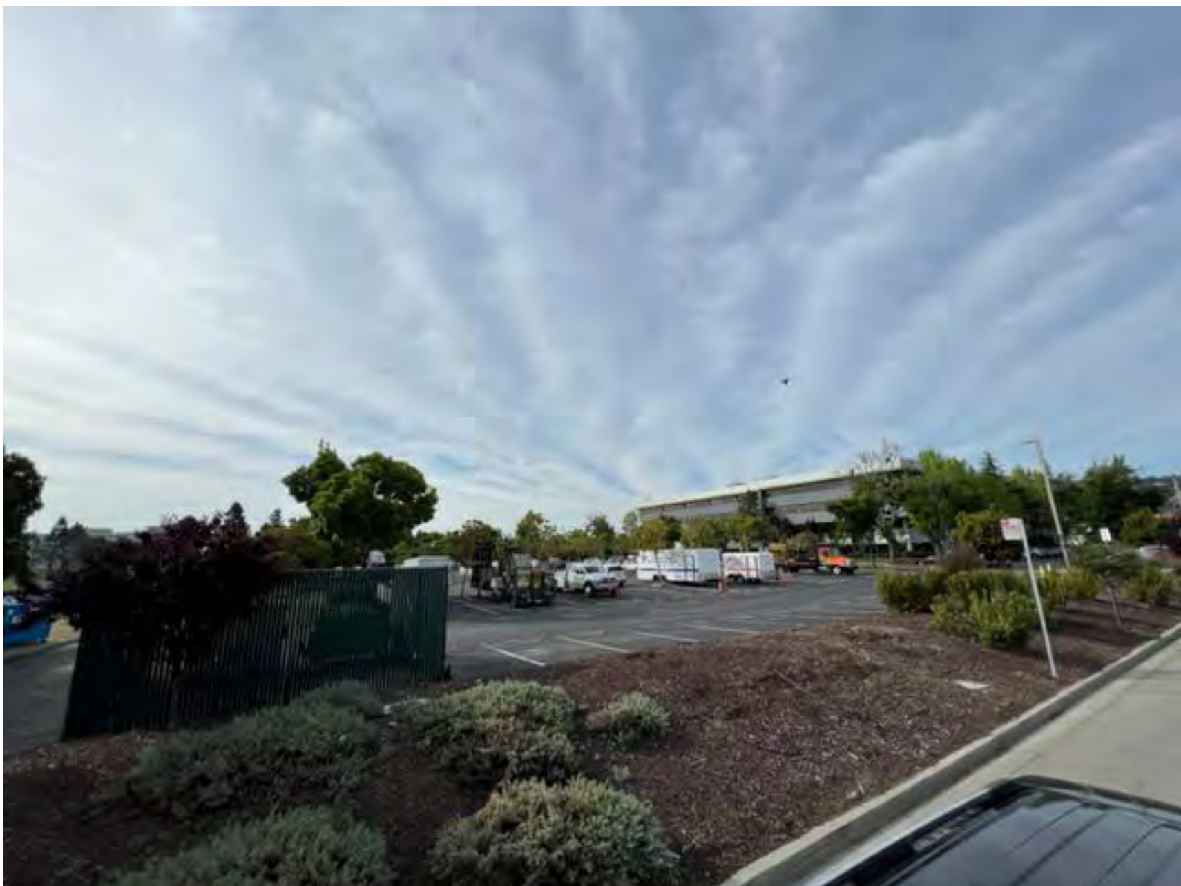
3 VIEW OF (E) 4 STORY BUILDING END OF SEM LANE @ BELMONT CREEK - LOOKING SOUTH
