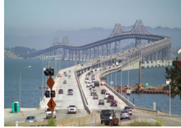
Richmond San Rafael Bridge Opened: 1956
