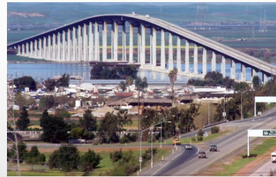
Antioch Bridge Opened: 1978
