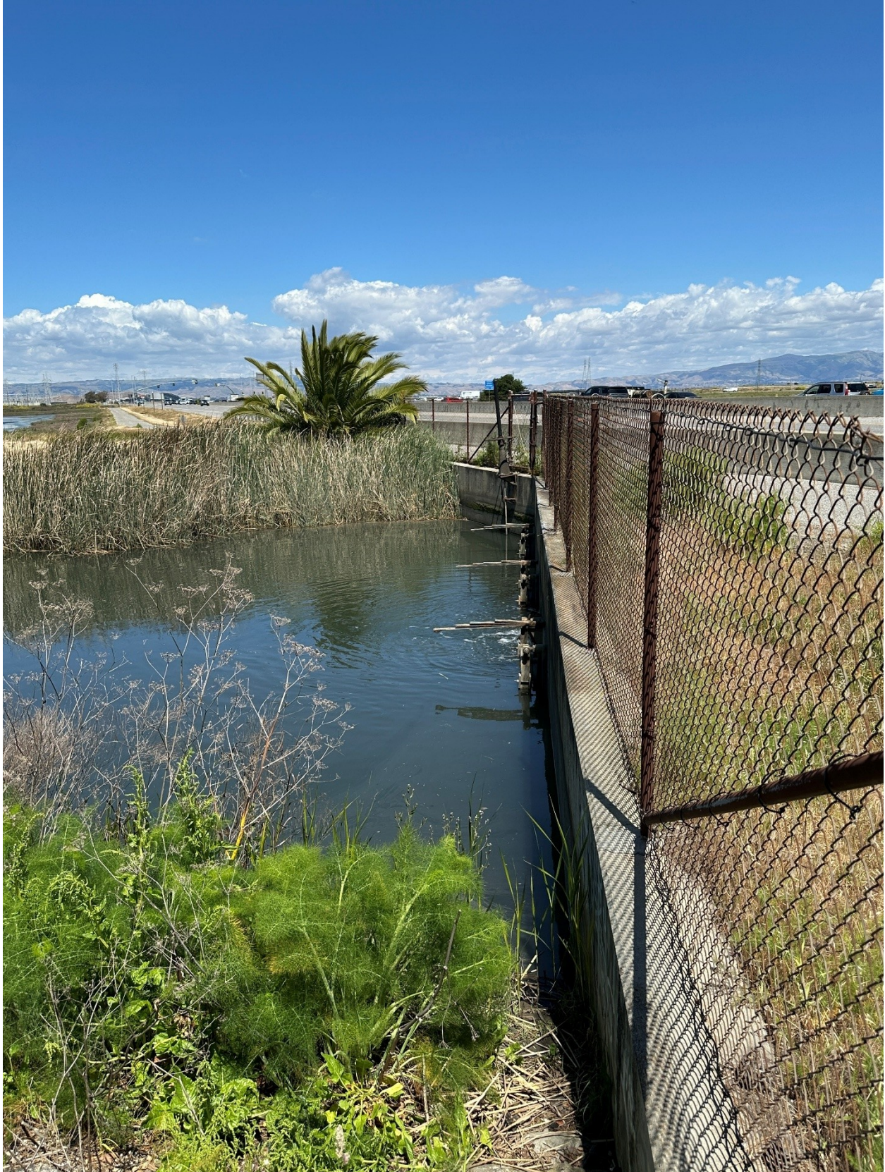
Figure 4-7: Ravenswood Pump Station Discharge Outfall
