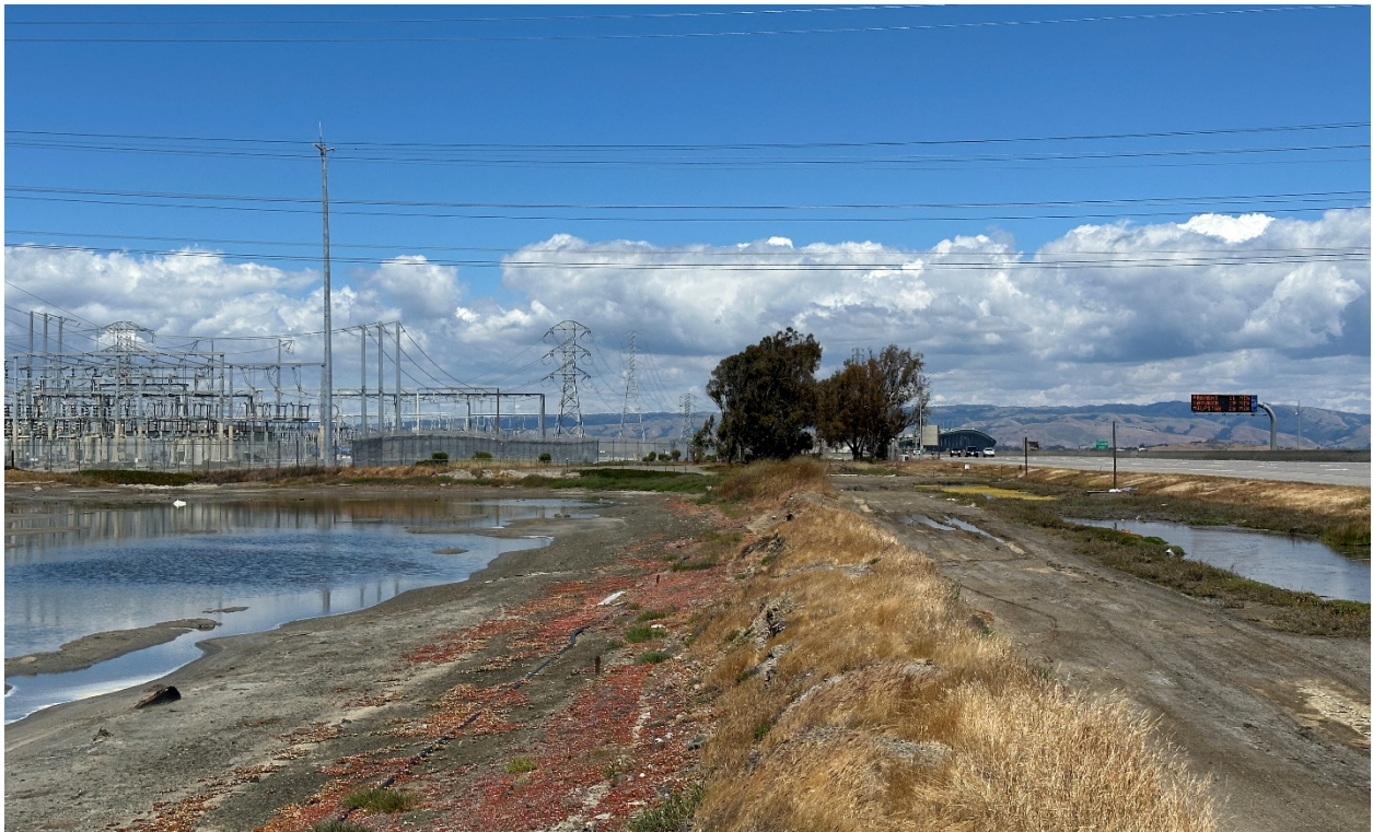
Figure 4-5: Near End of Substation and Marsh Restoration Reach Looking East
