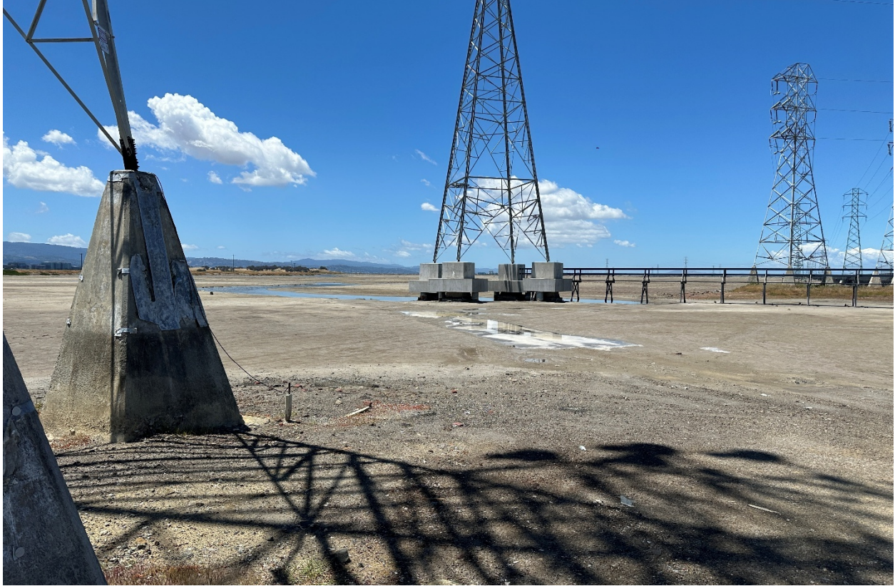
Figure 4-4: West of Substation near End of Substation and Marsh Restoration Reach
