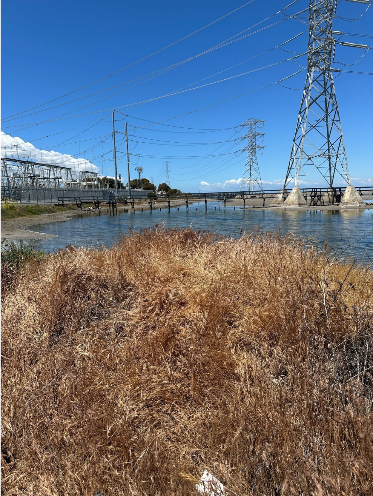
Figure 4-3: Transmission Lines at PG&E Substation
