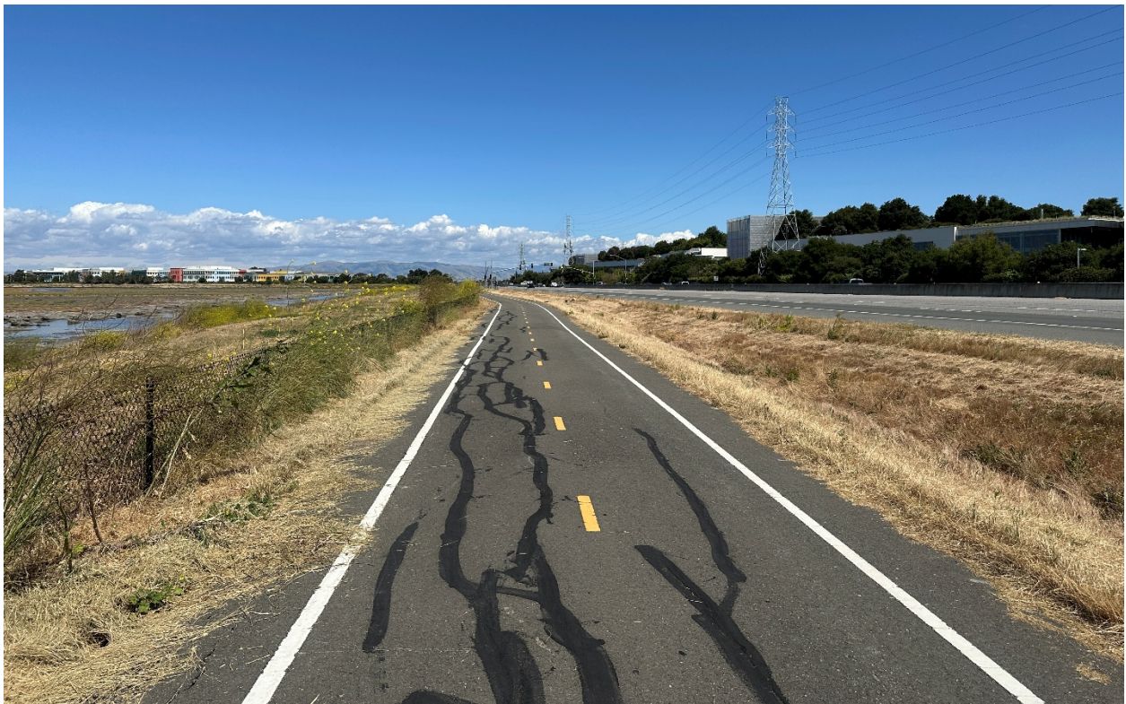
Figure 4-9: Bayfront Expressway Reach Looking East with Meta in Distance
