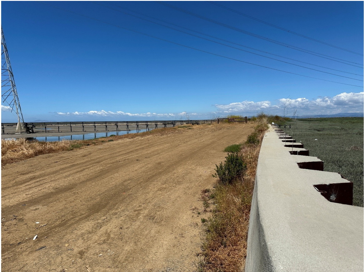
Figure 4-1: Near East End (Start) of Menlo Park SAFER Bay
