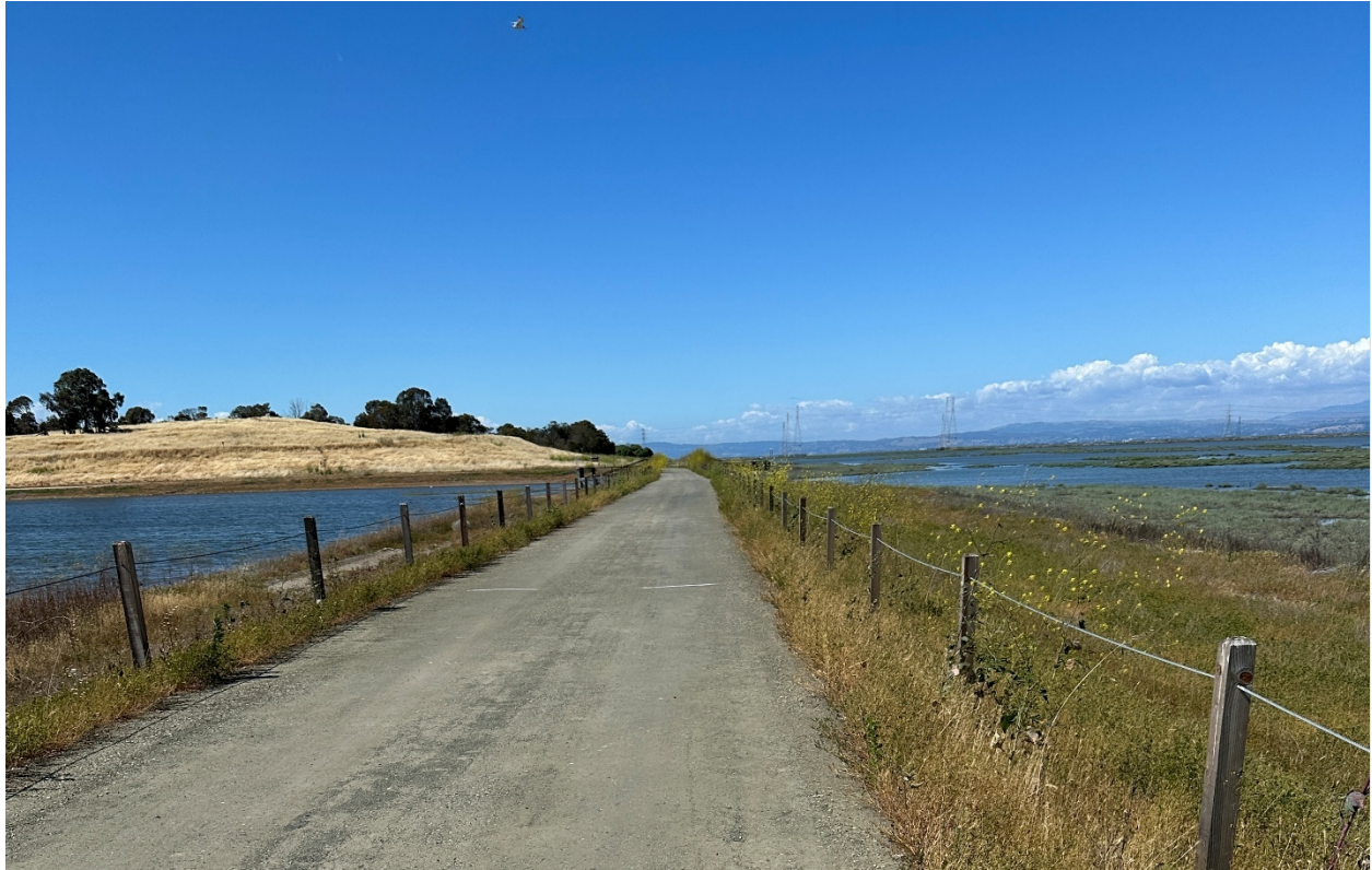
Figure 4-12: Levee Alignment Looking North Toward Bedwell Park
