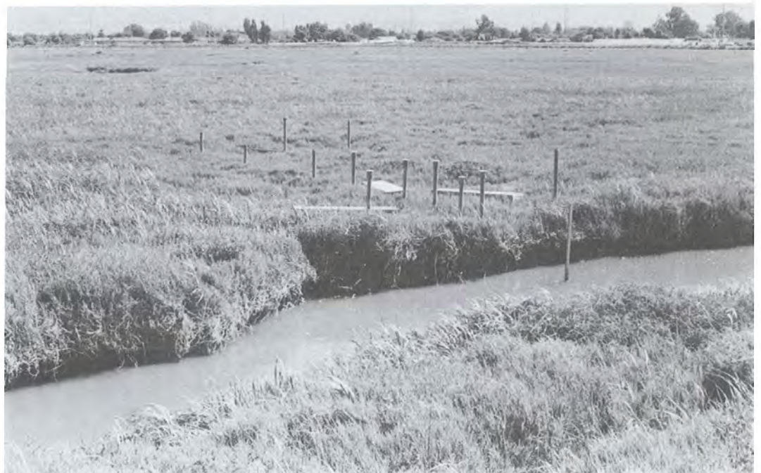
Plate 4. Piezometer set-up during high channel stage.
