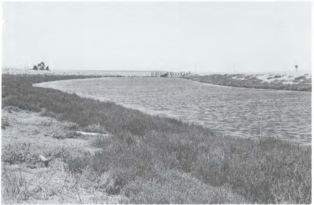
Plate 9. Dredged slough with bordering levees (looking northwest). Note tidal gate in background. Salicornia dominates the foreground.
