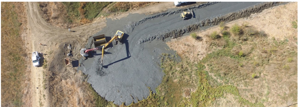
▲ Workers place a layer of sediment dredged from Novato Creek to raise the elevation of Deer Island in Marin County. Credit: Roger Leventhal
