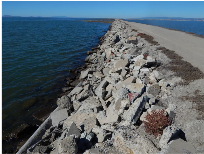
Concrete slab/rubble-armored bayfront levee south of fringing salt marsh/barrier complex.
