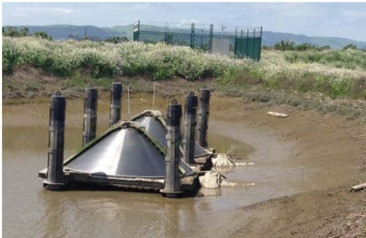
Figure 8-2. Example of Conical Fish Screen at Low Tide (Napa Sonoma Marshes Wildlife Area)
