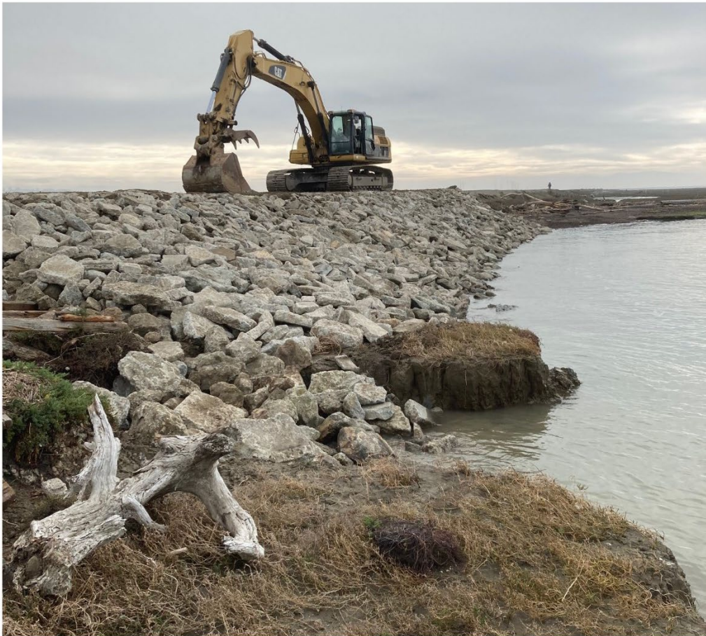
Figure 206. Riprap Placed on Outboard Side of Berm
