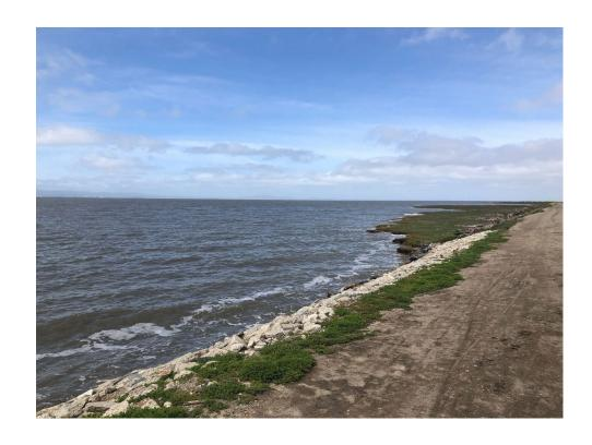
Outboard salt pond berm slope protected with repurposed concrete riprap.
