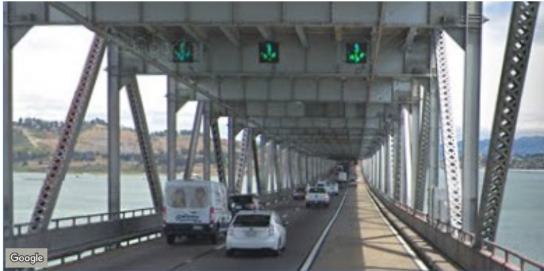
Figure 2-15: Electronic Lane Control Signs on Lower Deck
