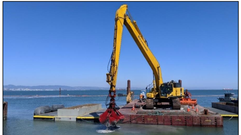
Example of offshore material dredging work
