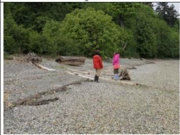
d) Weaverling Spit, Samish Indian Reservation; 1 of 4 large log drift sills within a 500-ft-long project in a highly degraded net shore-drift cell.
