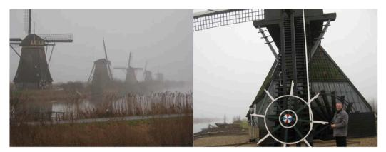
Figure 7. Many windmills built in the 18<sup>th</sup> century have been preserved, such as this impressive line of mills at Kinderdijk, which is a UNESCO World Heritage Site. Technology of such windmills is intriguing; the whole top can be turned following the wind direction.
