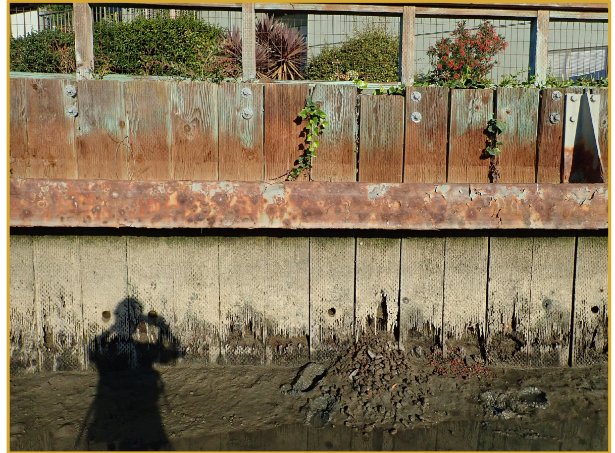
Typical Condition at Segment "B"
