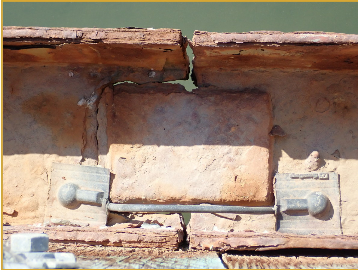
Typical Condition of Steel Wale
