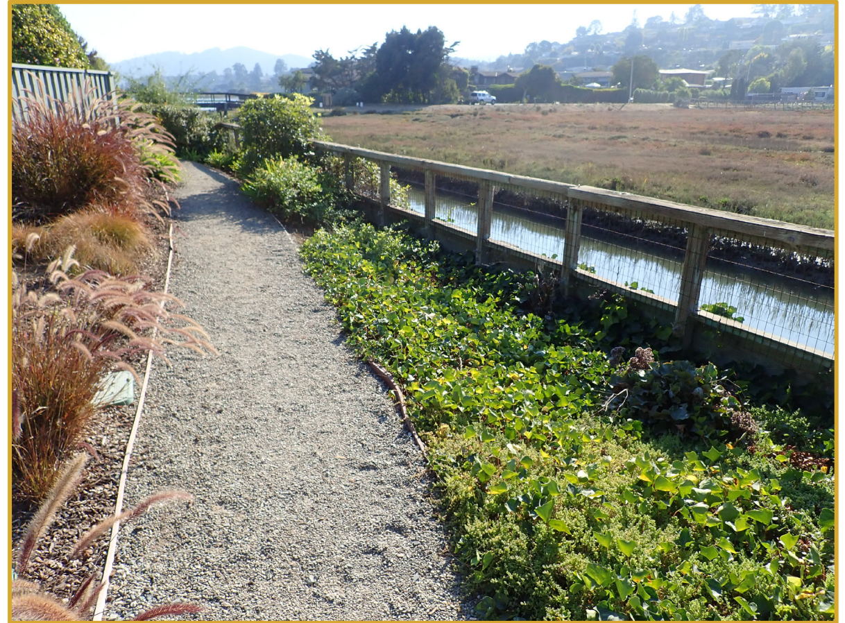
Typical View of Existing Grade at Top
