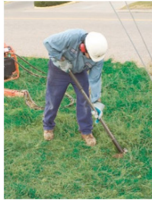
3. Pull the drive steel out of the ground.
