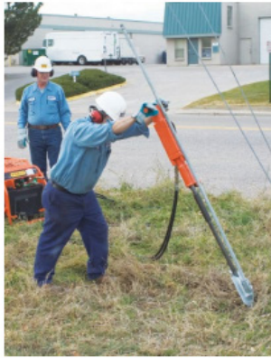
2. Insert drive steel into the anchor. Position and angle.
