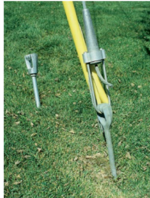
6. After removing the Load Locker, the eye is threaded to the end of the anchor rod. Now it's ready for guying.
