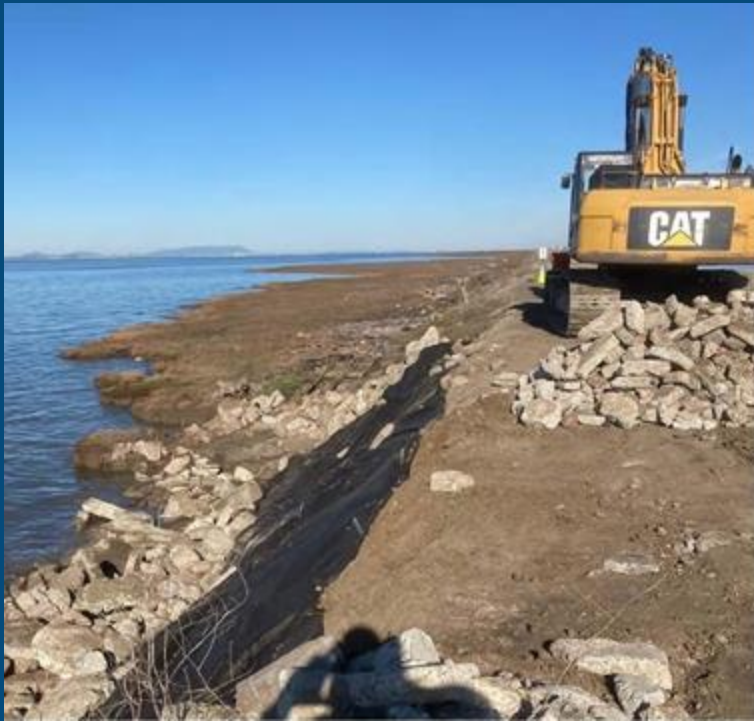
Photo of berm maintenance, from Draft EA, 2021
