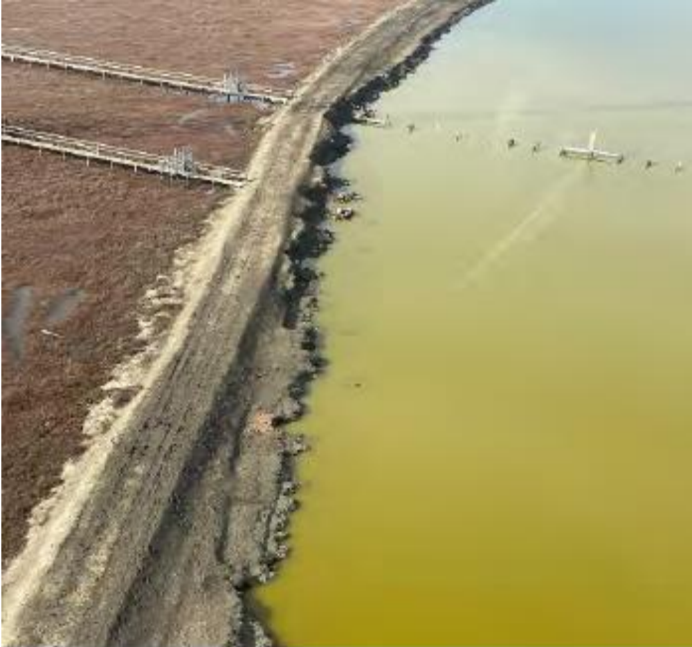
Salt pond berm photo from Cargill Maintenance Memo, 2021
